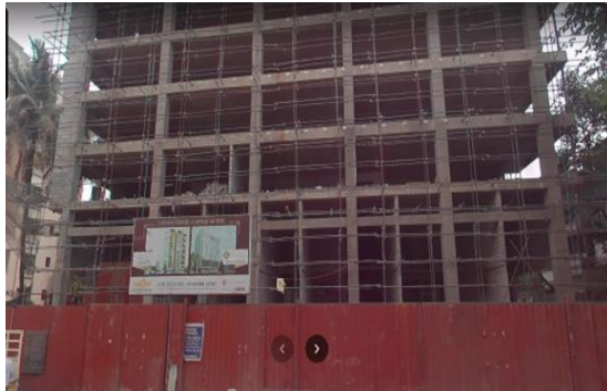
Redevelopment in progress
