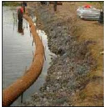
COIR LOG LAID ALONG THE WATER EDGE
