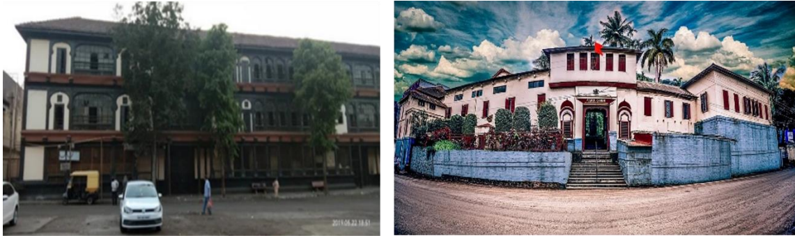
Figure 5: Rajwada Palace (Left) (Source: Author) and Adalat Wada (Right) (Source: https://commons.wikimedia.org/wiki/Main_Page )
