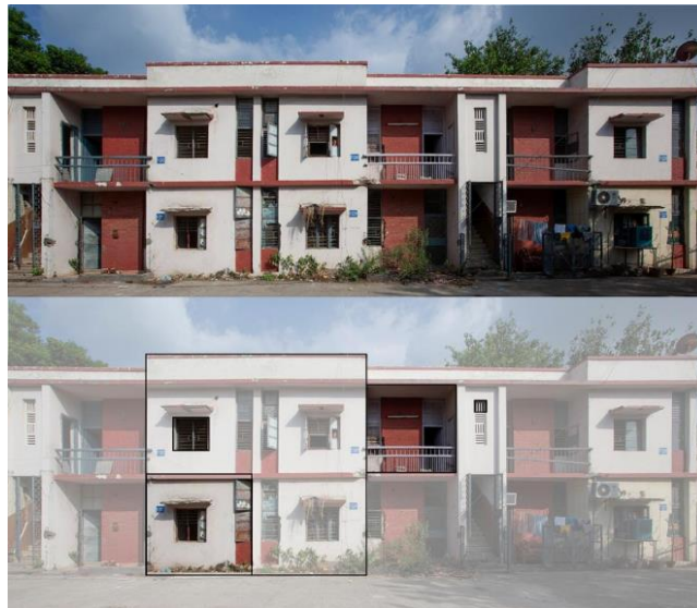
Figure 11: Rahman Type Flats' in June 2018 (Source: https://architexturez.net/file/36316932-1038890142947047-3247879643901984768-o-jpg )
