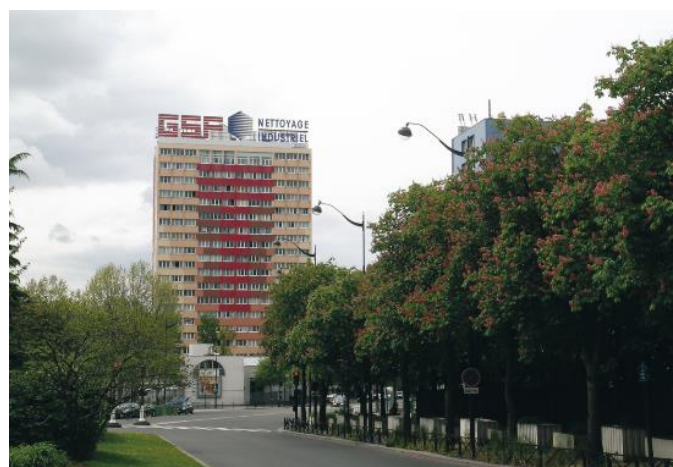
Figure 6: The Tour Bois le Prêtre (2011) – Before intervention (Source: https://metropolismag.com/profiles/lacaton-vassal-pioneered-strategy-saving-france-social-housing/ )
