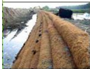
COIR LOG LAID AT SLOPE NEAR WATER EDGE
