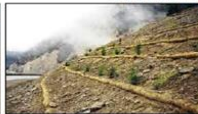
Figure 10 : Coir logs along the south edge of Charlotte lake :
