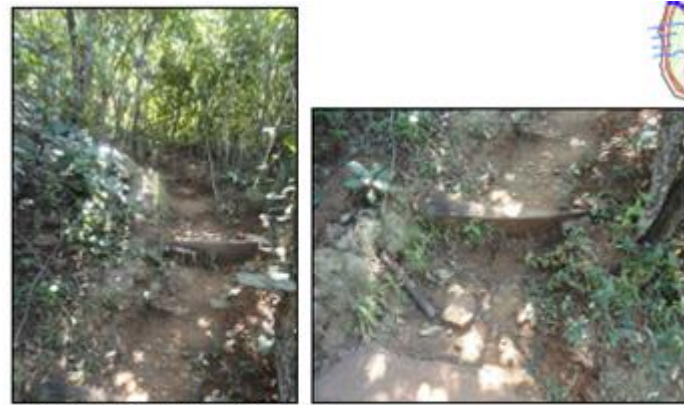
COIR LOGS LAID ON BOTH ROAD EDGES
