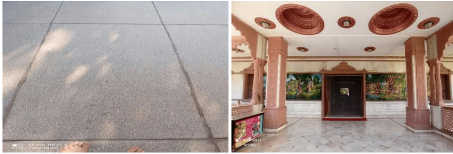
Figure 29: Concrete flooring of Radha Krishna (Left) and White marble flooring of Balaji temple (Right) (Source: Author)
