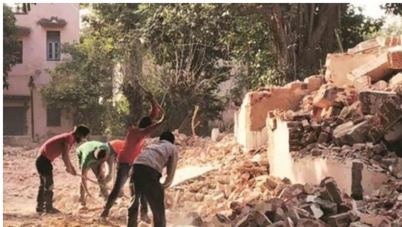
Figure 8: Demolition and tree-felling at Sarojini Nagar (Source: https://indianexpress.com/article/cities/delhi/activists-oppose-tree-felling-in-sarojini-nagar-nbcc-says-had-court-clearance-5532826/ )
