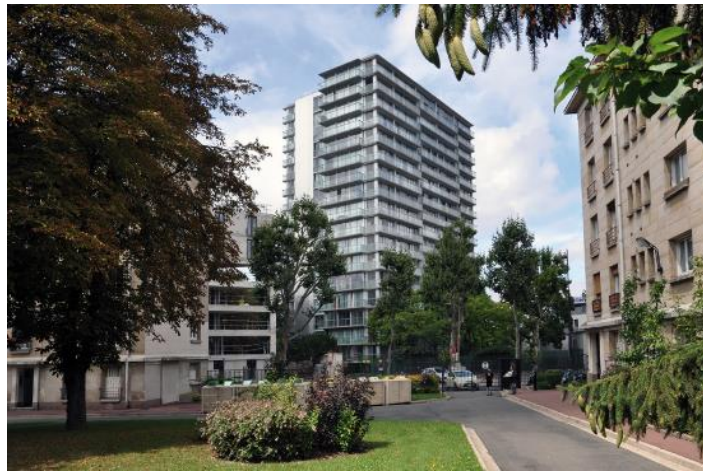
Figure 7: The Tour Bois le Prêtre (2011) – After intervention (Source: https://metropolismag.com/profiles/lacaton-vassal-pioneered-strategy-saving-france-social-housing/ )
