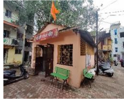
Figure 11: Enclosure of Community temple (Source: Author)
