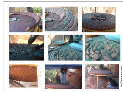
Figure 4. Refers to funicular shell roofs -construction techniques
