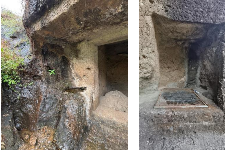
Figure 20, 21. Source – Author / At Kondivite caves Source – Author / water tank inside the niche at Kondivite caves
