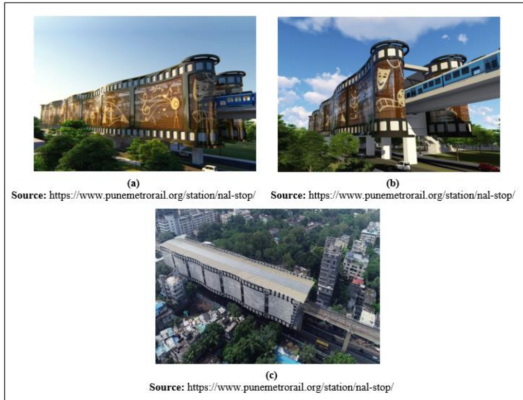
Figure 2: (a), (b) Architectural View of Nal Stop Metro Station; (c) Work Progress Update of Nal Stop Metro Station – September 2022
