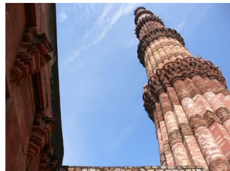
Figure 6: Qutub Minar showing horizontal carvings and vertical alternate angular and rounded grooves or flutings.
