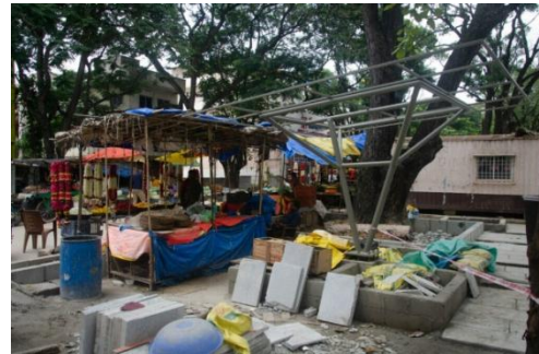
Figure 14: Installation of vendor infrastructure during the Gandhi Bazaar redevelopment
