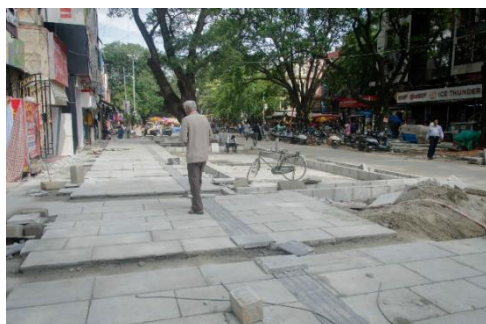
Figure 13: Redevelopment works at Gandhi Bazaar
