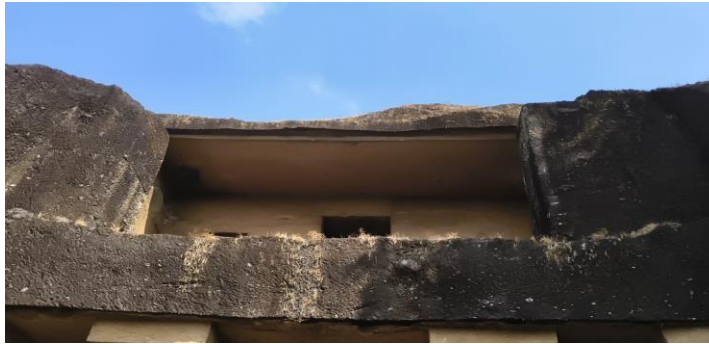
Figure 10. Source – Author / Drip moulding at cave no 1
