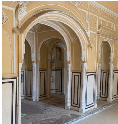
Figure 9 Use of lime plaster in Rajasthan architecture
