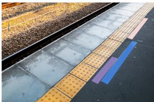
Figure 24. Braille system on ramps
